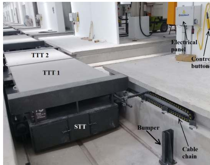
Figure 7. Transfer trolleys after installation
