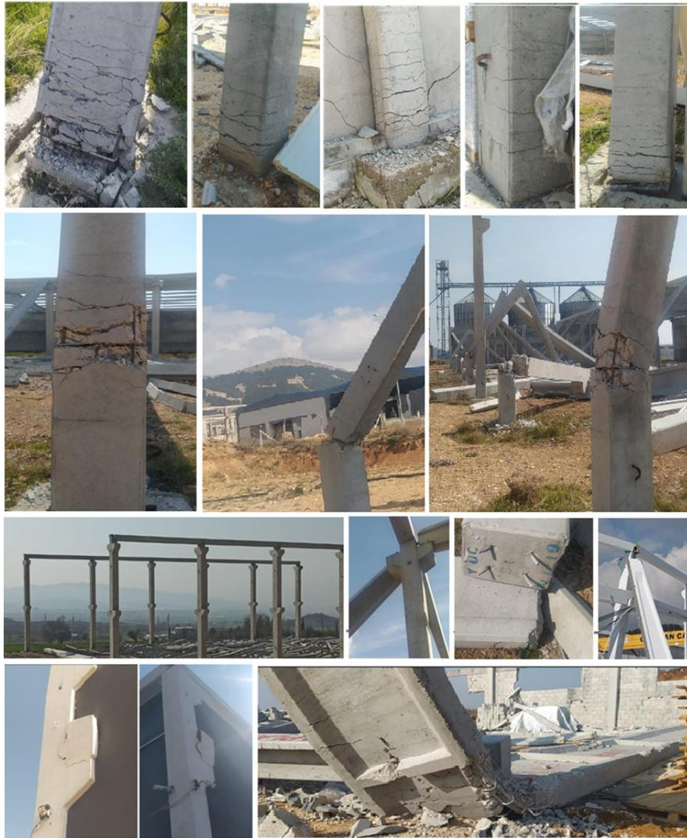
**Figure 2.** Common types of damage observed in precast RC structures.
