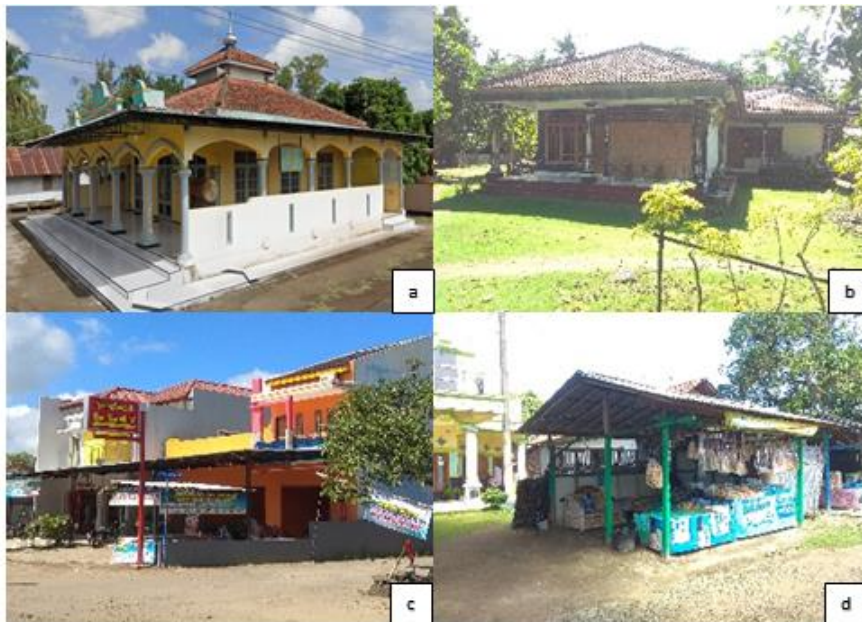
Figure 5. List of buildings in Jetis, (a) mosque, (b) residents' houses, (c) stores, (d) temporary buildings.
