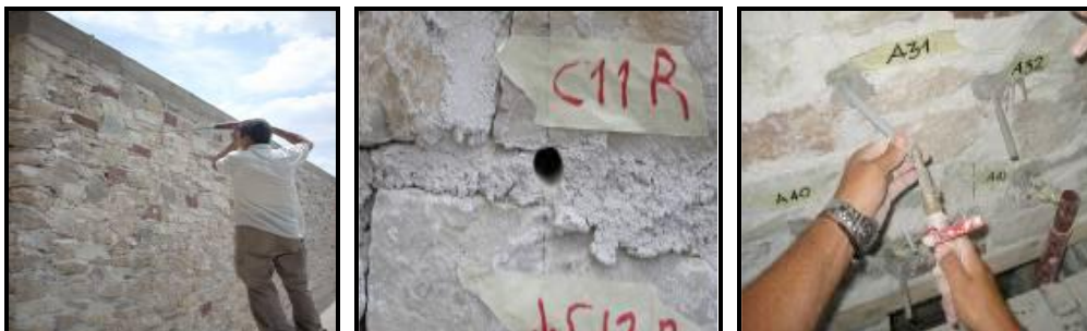
Fig. 5. Grout injection procedure, drilling holes in mortar joints and fixing
