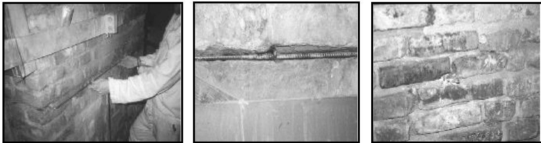
Fig. 7. Execution stages in the case of reinforced re-pointing performed
