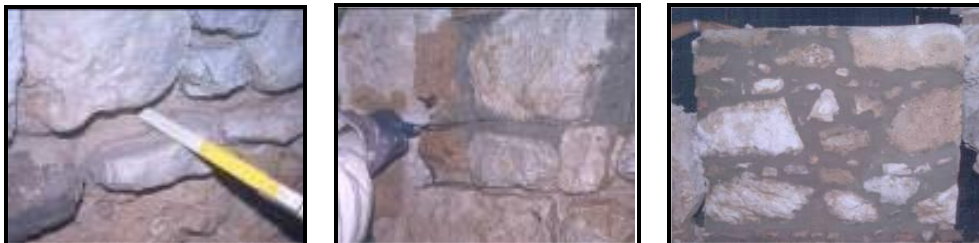
Fig. 1. Grout injection procedure, drilling holes in mortar joints and fixing
