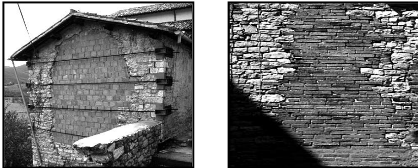
Fig. 9. Masonry replacement intervention
